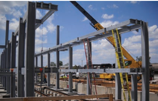
Steel erection for Locomotive Wash Facility - Bellevue, Ohio
